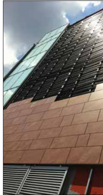
Hyatt Place Hotel Ventilated Rainscreen
